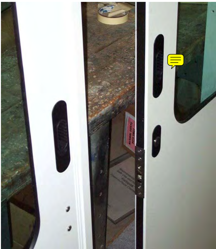
ASTRAGAL ON PASSIVE DOOR AND MOBELLA LOCK ON ACTIVE DOOR VIEWED FROM OUTSIDE
