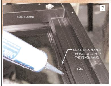
AFTER POCKET AND SILL BOTTOM ARE CAULKED, INSTALL FIXED PANEL BY INSERTING TOP OF PANEL INTO HEADER AND SLIDING PANEL FULLY INTO JAMB POCKET OF FIXED JAMB. USE A RUBBER MALLET TO SEAT FULLY INTO POCKET.
