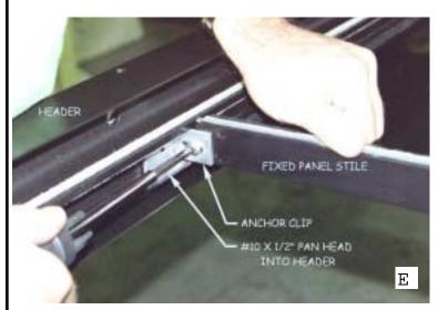
ANCHOR CLIP COMES INSTALLED ON FIXED PANEL.
